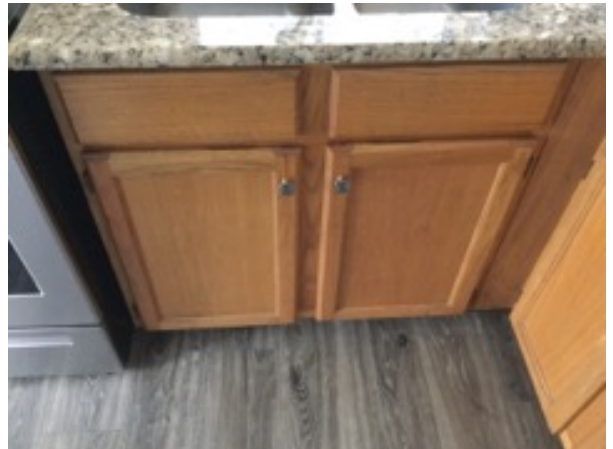
Cabinet Under Sink
