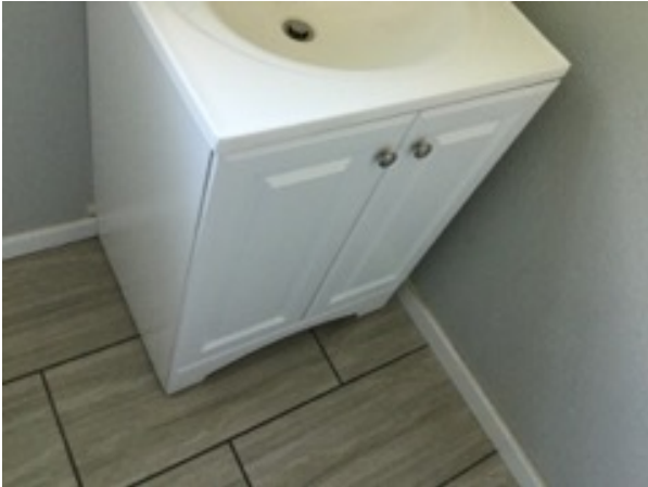
Cabinet Under Sink
