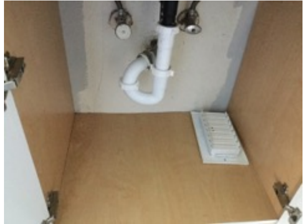
Cabinet Under Sink
