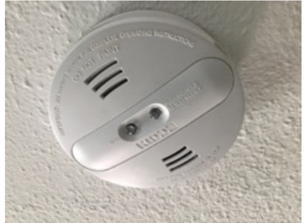
Smoke Alarm - Technician installed new battery.
