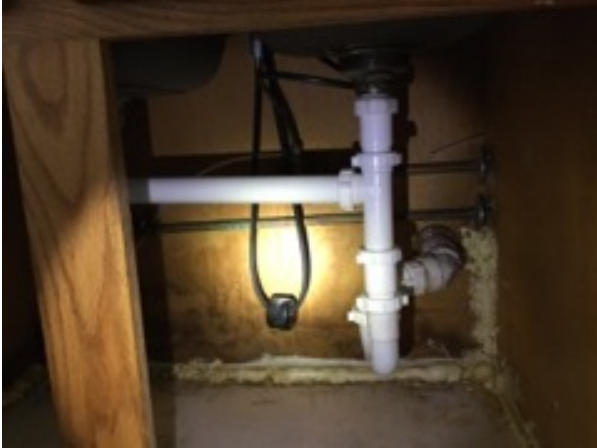
Cabinet Under Sink
