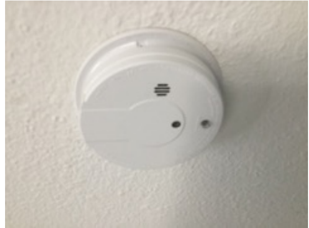
Smoke Alarm - Technician installed new battery.
