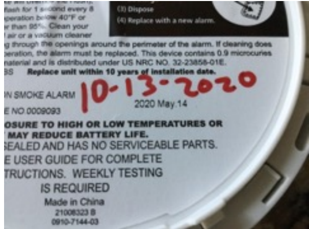
Smoke Alarm Installed (DATE)
