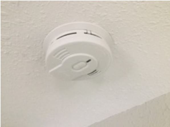
Smoke Alarm Installed
