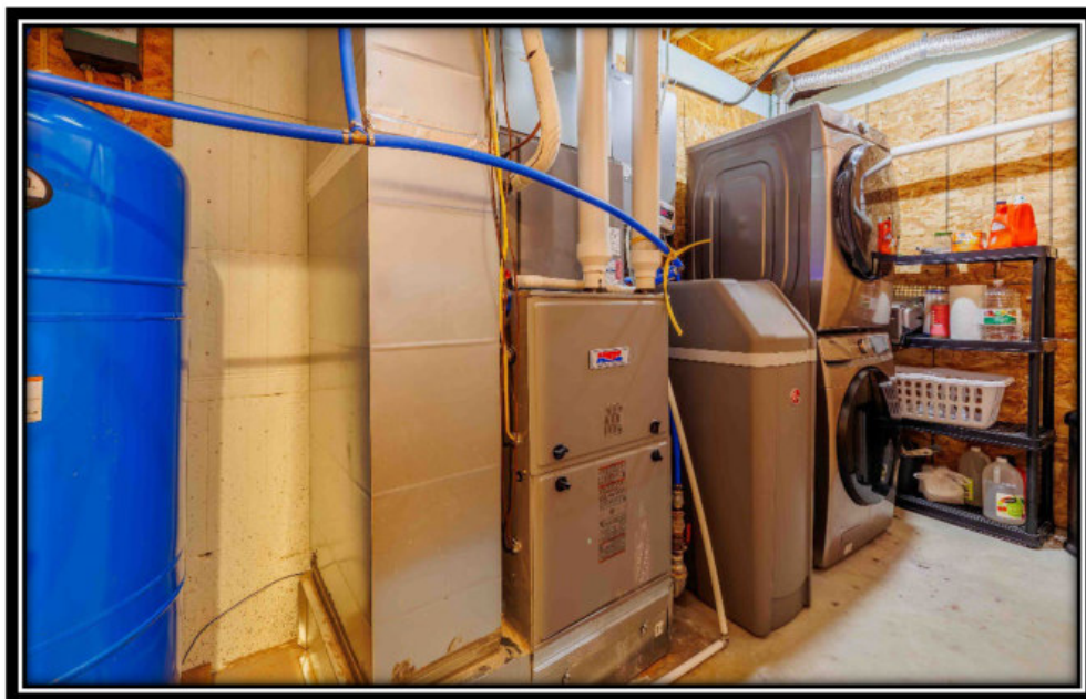
Laundry Utility Room
