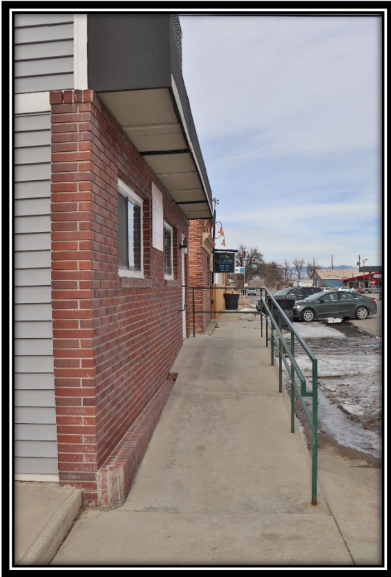
Front of Building to Salon with Ramp
