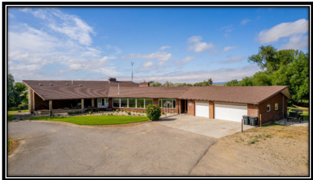
Exterior Front Entrance to the Home
