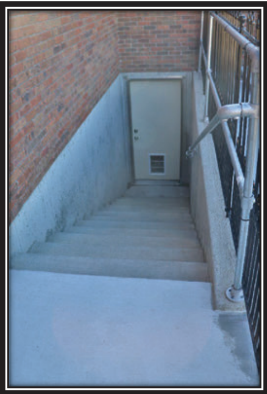
Exterior Entrance to Basement
