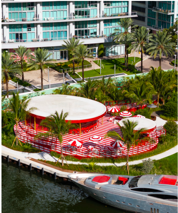
The Faena Residences Miami tower is under construction, but a temporary dock set-up is already built. ORIOLE TARRIDAS PHOTOGRAPHY
