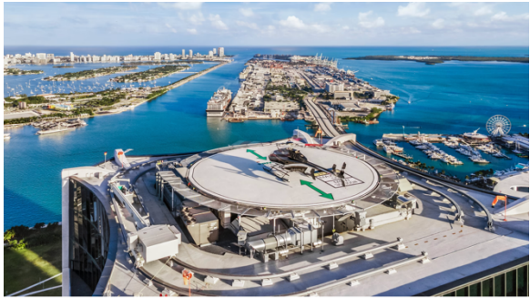
The rooftop helipad at One Thousand Museum. ONE THOUSAND MUSEUM
