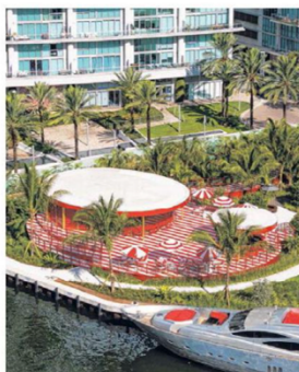
The Faena Residences Miami is under construction, but a temporary dock setup is already built.
