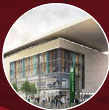
Kaiser Permanente Medical Building
